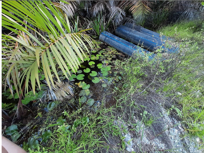
Photo 5. Good hydrological connectivity and no evidence of adverse impacts - culverts allowing exchange of water across a road
