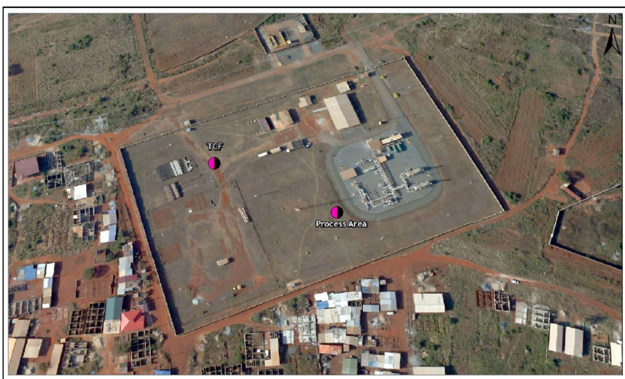
Figure 5: Aerial view of the Tema Regulating and Metering Station
