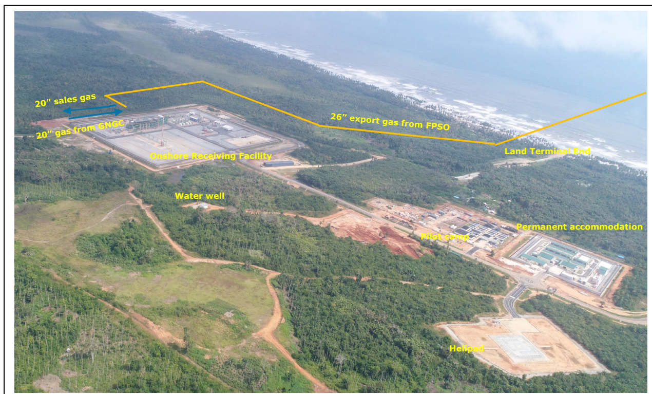
Figure 2: Aerial photograph of the Onshore Receiving Facility (October 2019)
