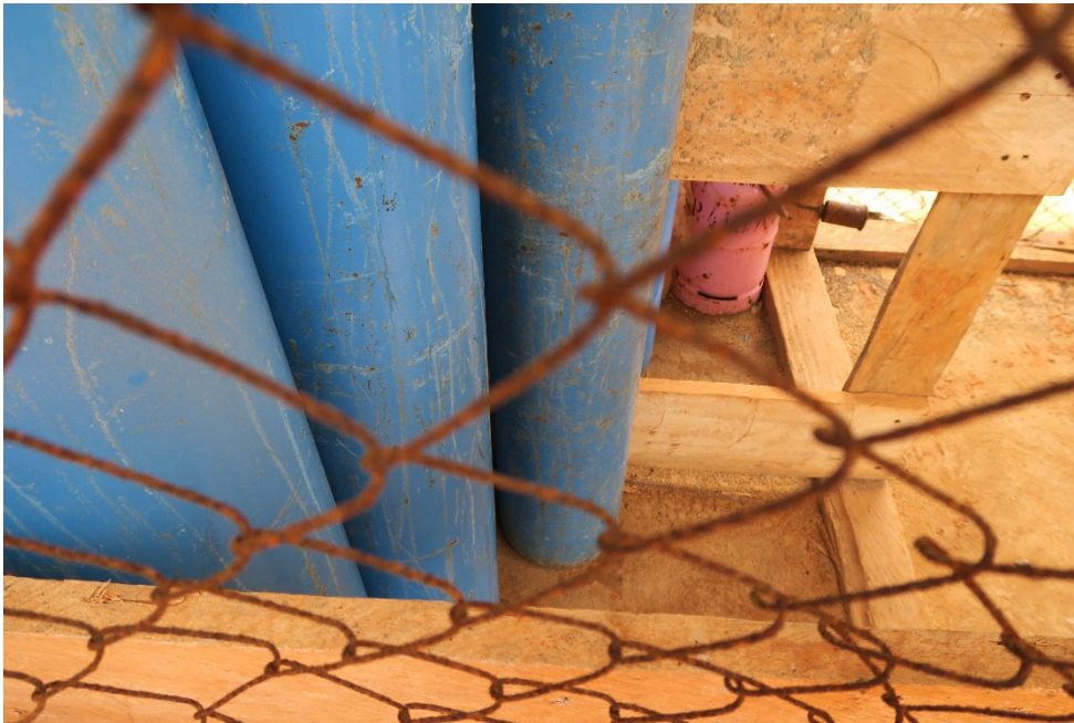
Photo 17. Compressed gas cylinders in a locked area but individual cylinders were unsecured
