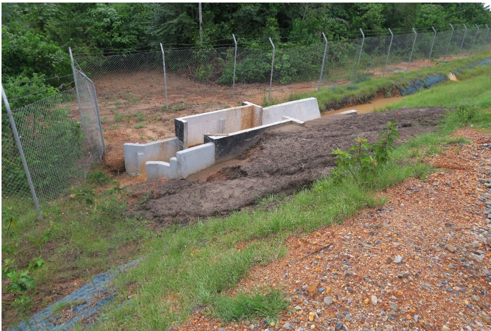
Photo 12. New sediment trap(s) installed to reduce sedimentation of receiving water bodies
