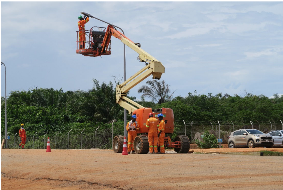
Photo 4. Good Safety practice – use of PPE, harness and HSE presence (indicated by red hard hat)
