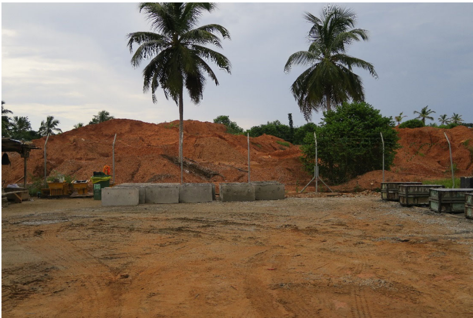
Photo 18. Large amounts of stockpiled earth from the permanent accommodation construction area
