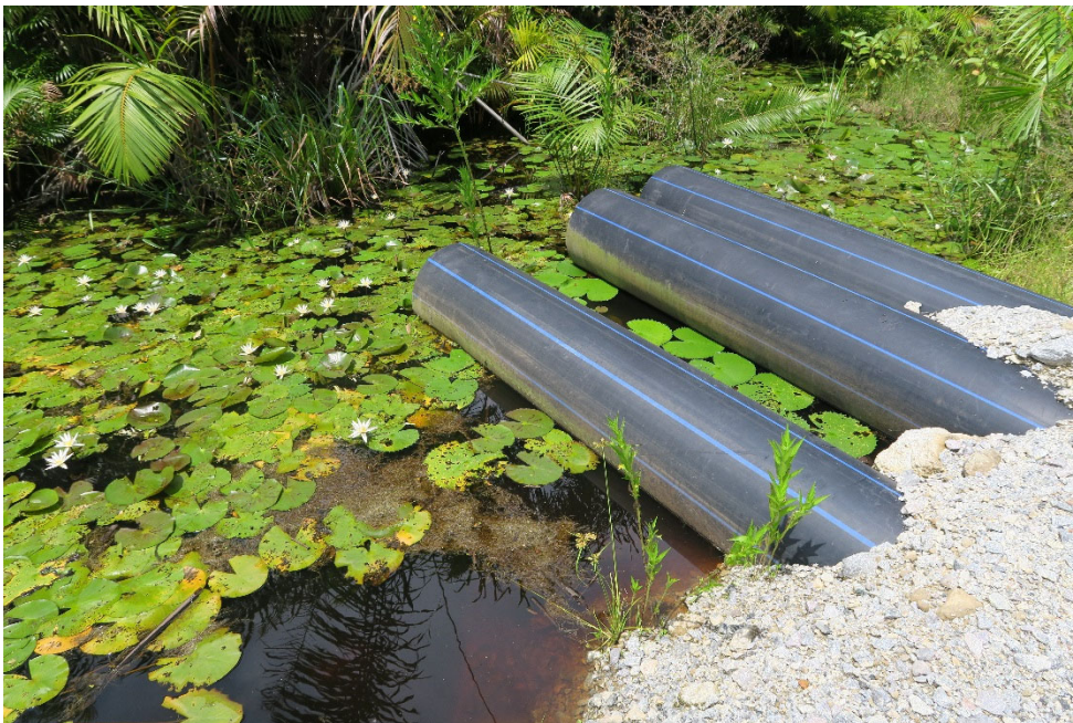
Photo 10. Exposed pipes intended to maintain hydrological connectivity of swamp area
