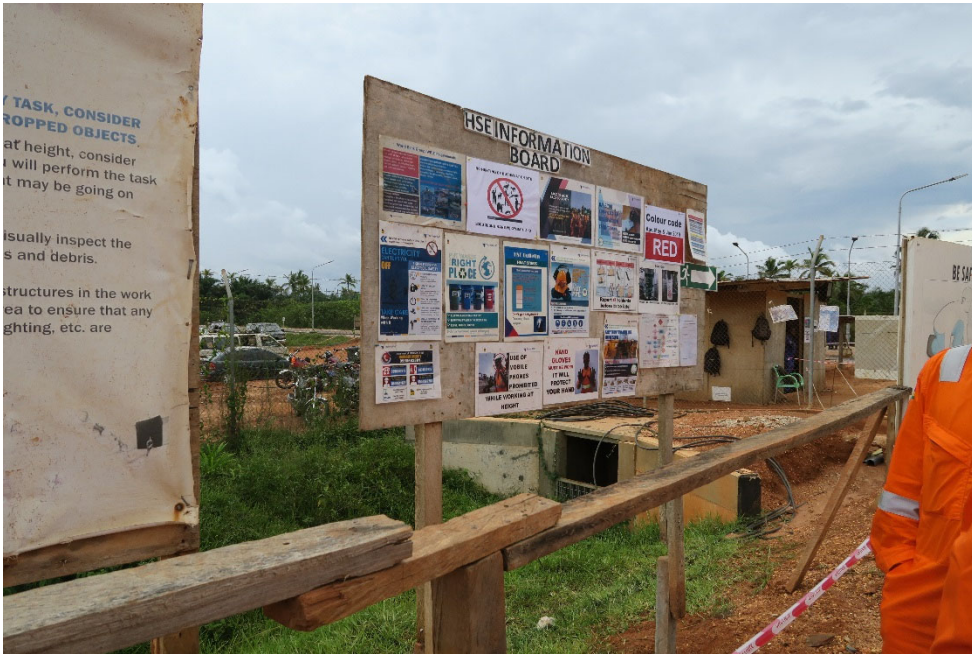
Photo 13. HSE signage at the permanent accommodation construction area
