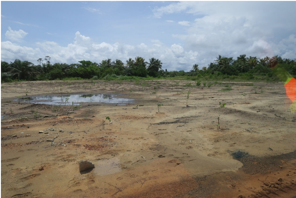
Photo 9. Reinstatement of area used to stockpile topsoil
