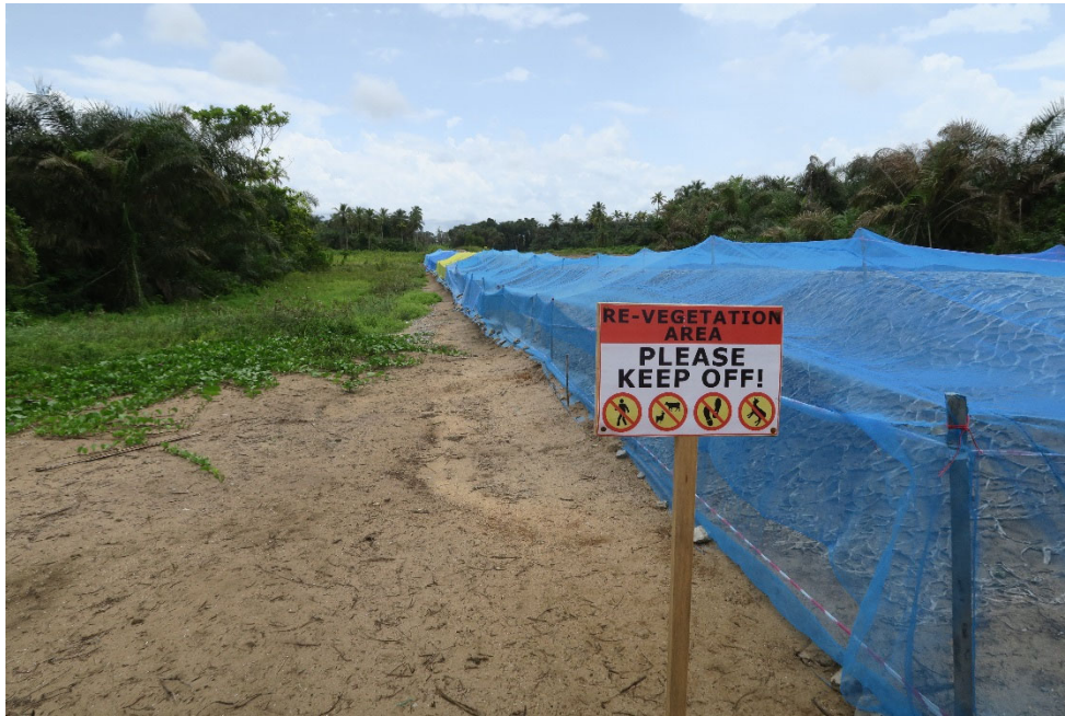
Photo 7. Reinstatement of pipeline bund – use of geotextile, seeding and plastic mesh to prevent erosion and deter invasive species
