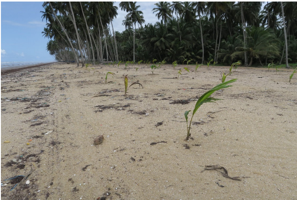
Photo 6. Reinstatement of beach area following post lay trenching of pipeline – coconut saplings
