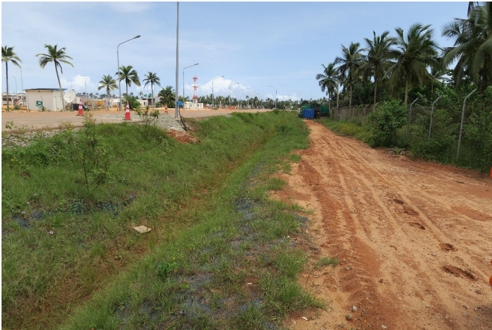
Photo 3. Drainage channels – vegetated to reduce erosion and sedimentation of receiving waters
